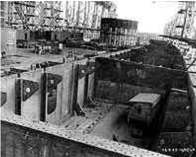
Incomplete hull, looking aft, at the New York Shipbuilding Company shipyard, Camden, New Jersey, 8 March 1922. Construction had been suspended, pending her conversion to an aircraft carrier. Note barbette structure resting on blocks on her deck.
