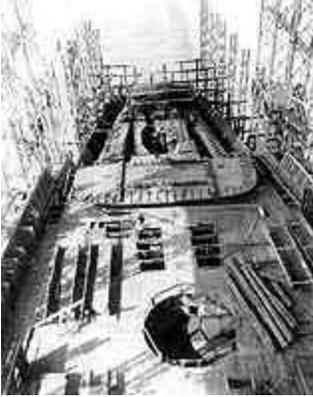
Incomplete hull, looking forward, at the New York Shipbuilding Company shipyard, Camden, New Jersey, 8 March 1922. Construction had been suspended, pending her conversion to an aircraft carrier. Note barbette structures resting on blocks on her deck.
